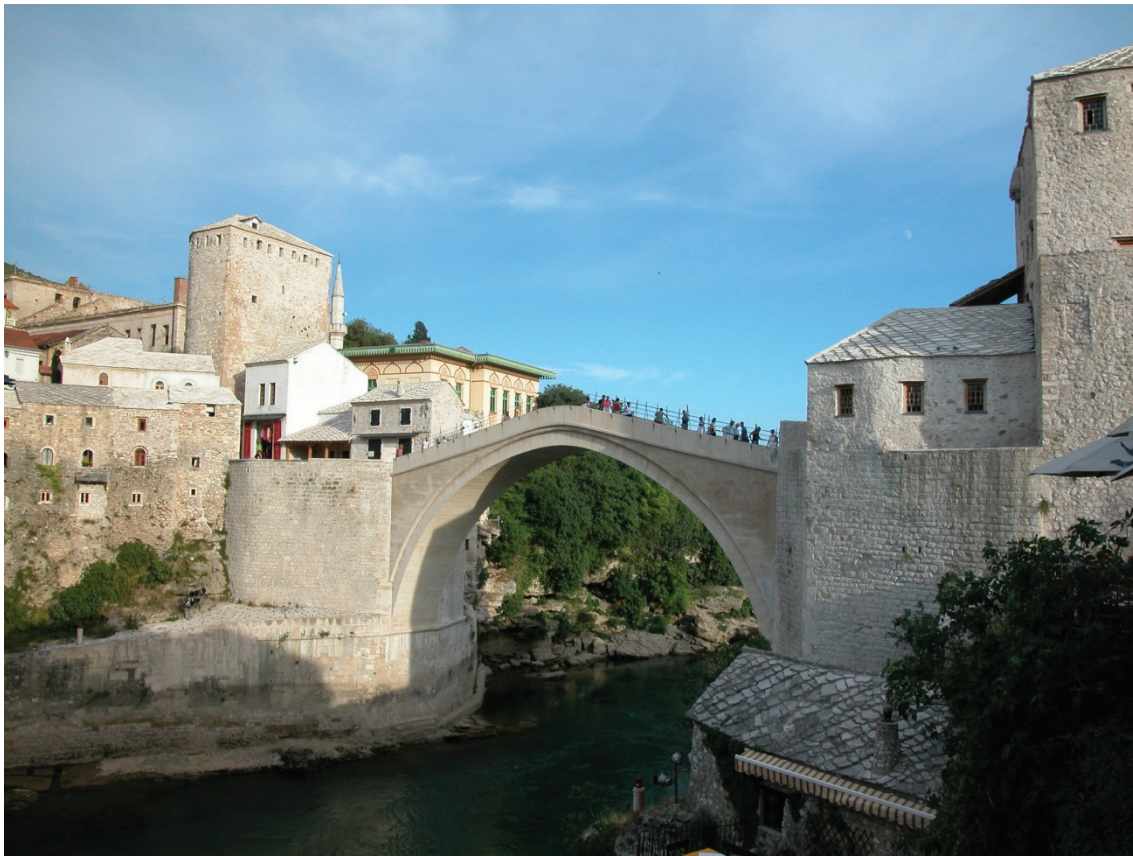
Figure 1. Photo of the rebuilt Stari most (Old Bridge).
