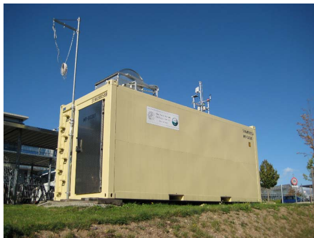
Fig. 1. Picture of the MPI-BGC FTIR container at its preliminary location close to the MPI-BGC in Jena.
