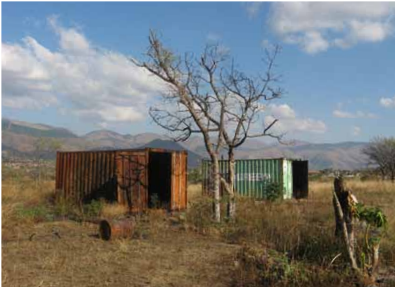
Photo 9: Burnt storage containers
