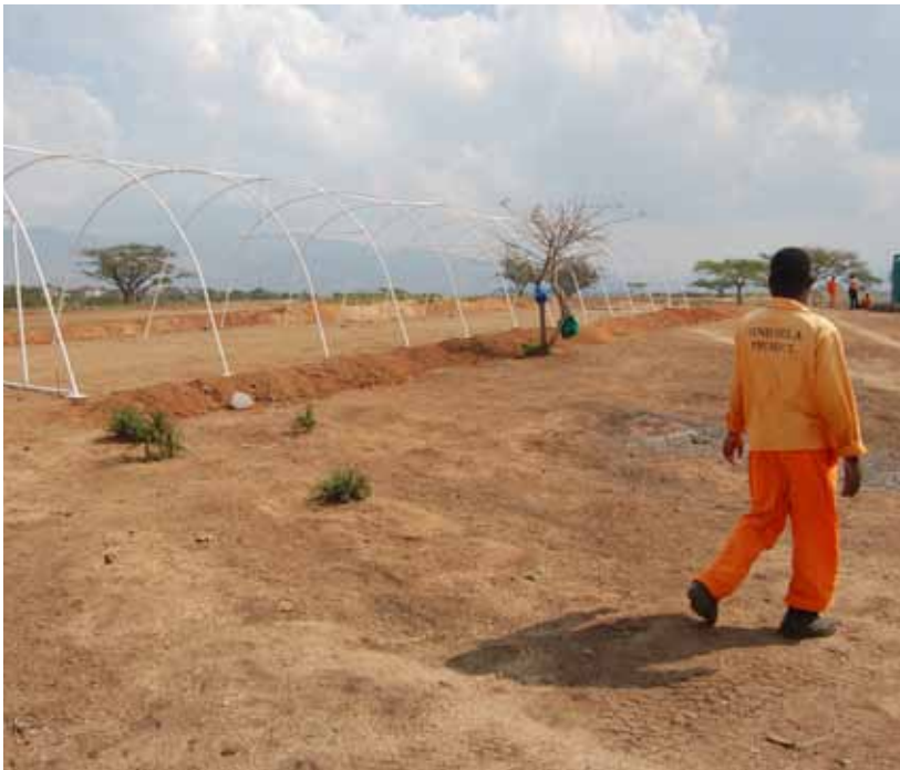
Photo 19: The new greenhouse construction
