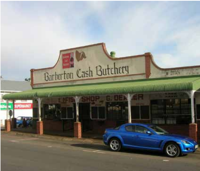
Photo 2: A historic building in Barbarton
