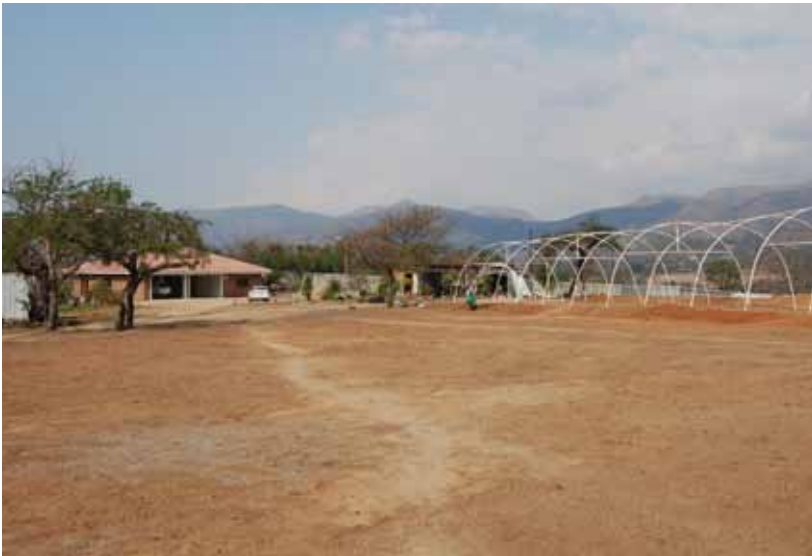
Photo 17: The new office building and a greenhouse construction
