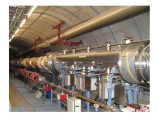
**Figure 29.** Kicker bypass in the HERA tunnel (West left 200 m). The bypass will be installed in the middle of the experiment connecting the two dipole strings of ALPS-IIc and pass the magnet current and the cryogenics around the optical setup.
