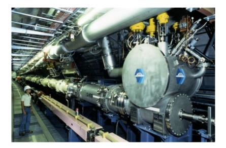
Figure 33. Cryogenic feed box for an octant of superconducting magnets at HERA.
