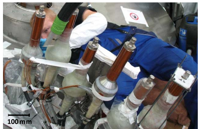
Fig. 10. Insulation of the last joints at the module section area
