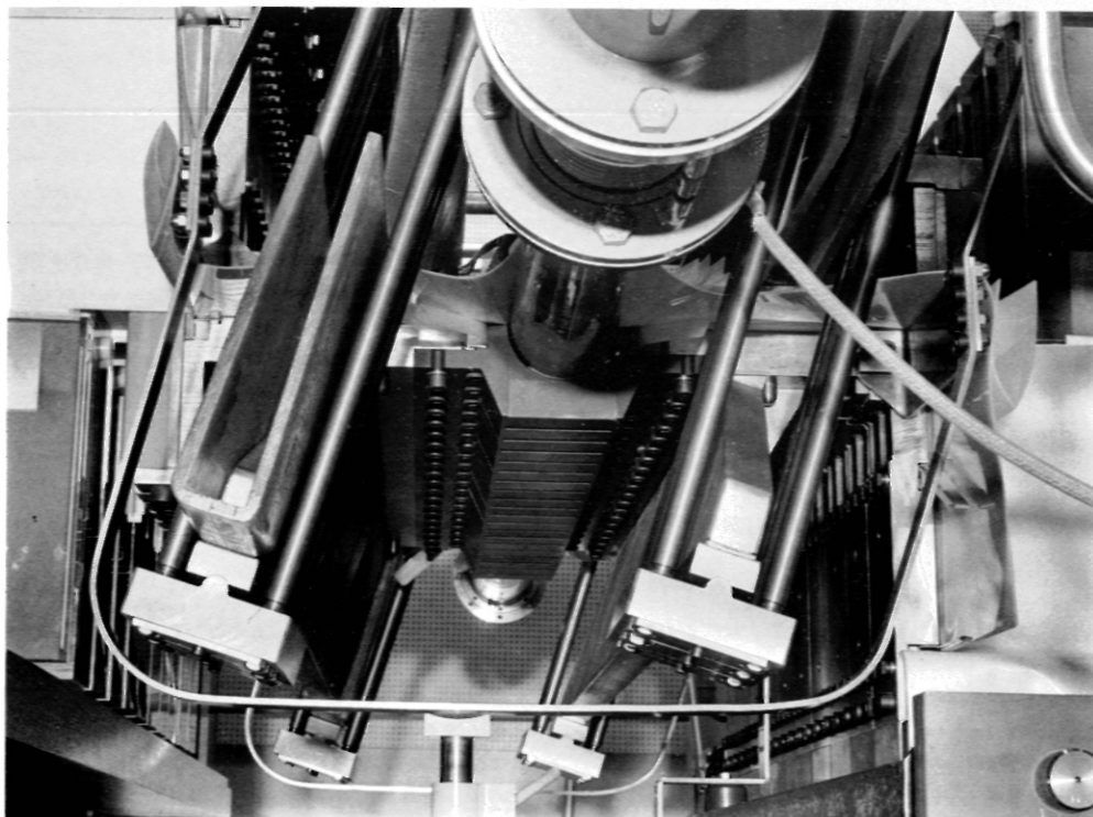
P 129 500 kJ - Theta - Pinch Isar II Coil, main collector with spanning
