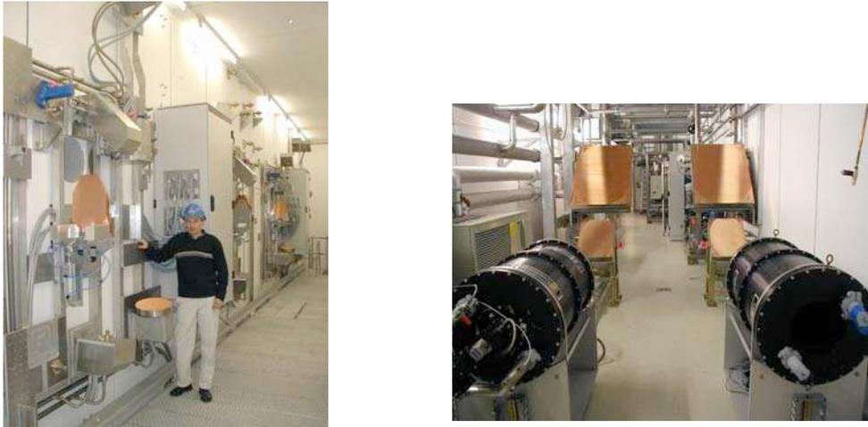
**Fig. 2.** Single beam mirror modules (left) and multi beam waveguide (right).
