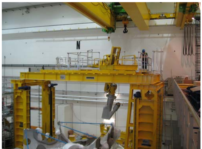
Figure 18: The port assembly bridge (inner and outer tower and upper cross-beam).
