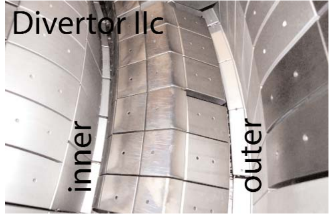
Figure 18: View of the new full W divertor
