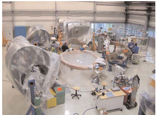
Figure 29: Preparation of coils and plasma vessels
