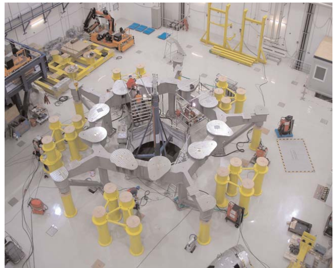
Figure 33: The machine base in the torus hall was delivered as planned
