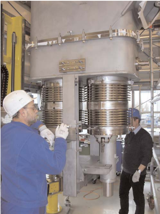
Figure 14: Assembly trial with CL-dummies and dome sections.
