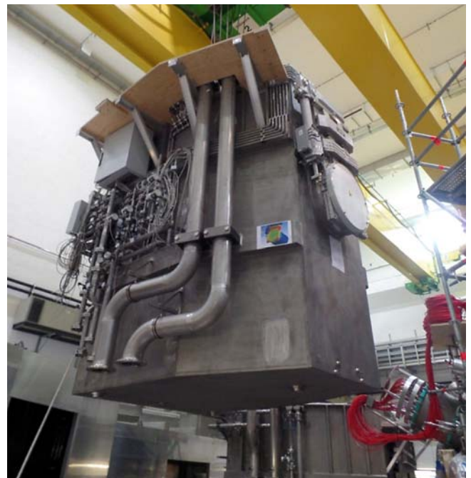
Figure 33: NBI-Box 21 being lowered into position on its support structure in the torus hall. The pipework completed in the NBI pre-assembly hall as well as some of the cabling for the control/DAQ system can be seen.
