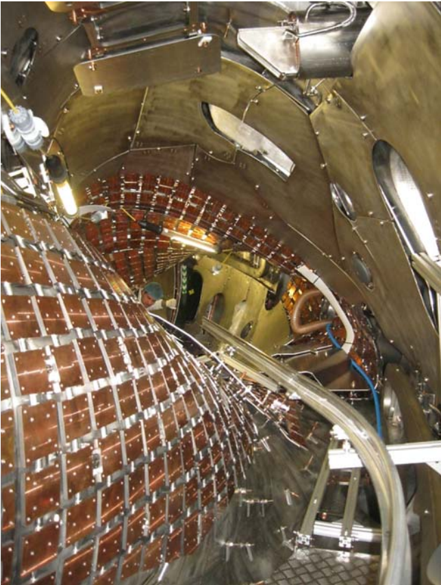
Figure 7: The in-vessel setup for OPI.1. Temporary assembly equipment like the rail system, steps, cables, hoses is removed.
