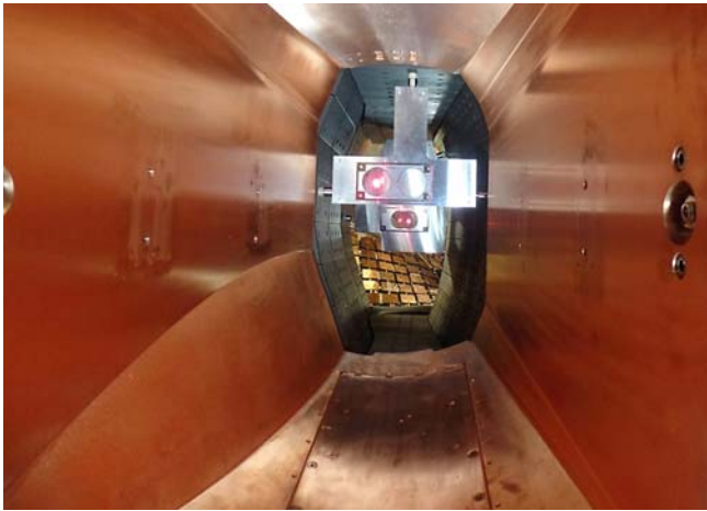
Figure 34: View from inside of bellow scraper in AEK21: two targets are used to align the NBI beam with respect to the duct. Strike points of laser beams for NBI-Box alignment are visible. This picture also shows that the KiP structures including carbon/CFC tiles are installed in the NBI duct.
