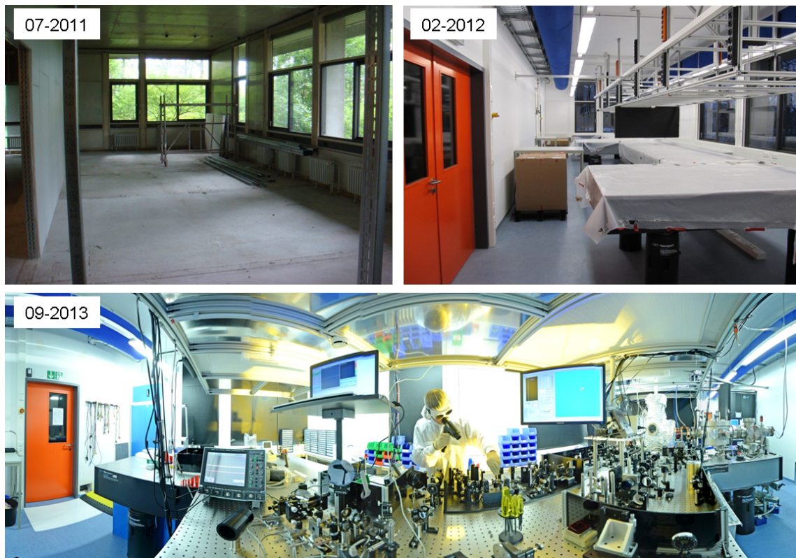
Figure 2.2: Pictures of the new laboratory that was built for the 100 keV electron diffraction experiment. The first picture was taken in July 2011 and shows only a construction area; in February 2012 the optical tables arrived and in September 2013 the first diffraction measurements were made.
