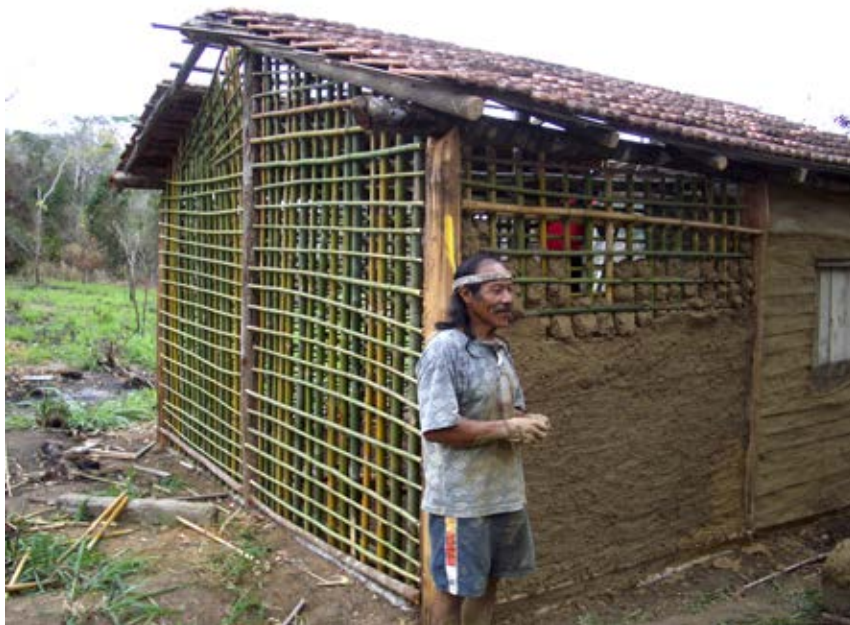
Figure 23.3: The former chief Jonas explains how to use raw materials (mud and bamboo) to build a more traditional Indian house, which has a lesser impact on nature. (Photo by Silva, 2008)
