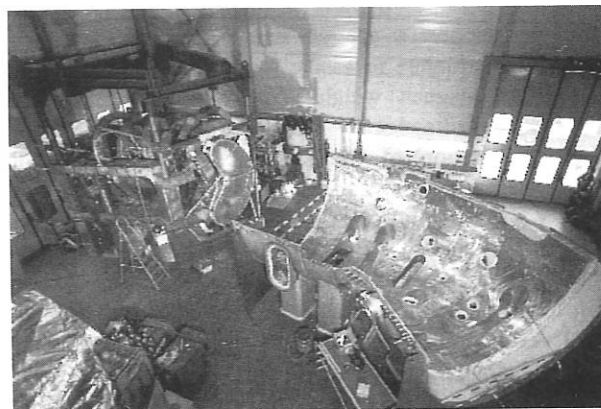
FIG. 2: Lower part of the cryostat vessel (in front) and the basic unit comprising the plasma vessel, the model magnets, the support structure and the insulation.
