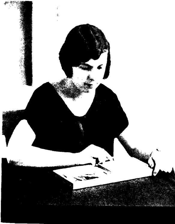
FIGURE 7. WORKSAMPLE NO. 17, TWEEZER DEXTERITY Apparatus used in measuring the tweezer dexterity of factory workers who apply for positions requiring the use of tweezers, such as miniature instrument assembly or glass blowing.
