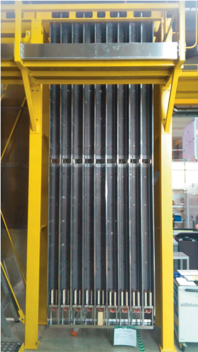
Figure 13: Assembly of the titanium sublimation pumps in the storage scaffold.
