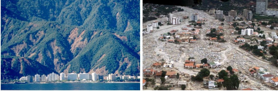
Figure 1.2: Example of major mudslides in Venezuela (dark brown color in the left image, light brown color in the right image). The disaster is known as the Vargas tragedy in December 1999, causing many deaths and extensive damage to towns, cities and infrastructure. Heavy rain triggered thousands of shallow landslides that evolved into debris flows. Images from Wikimedia Commons.
