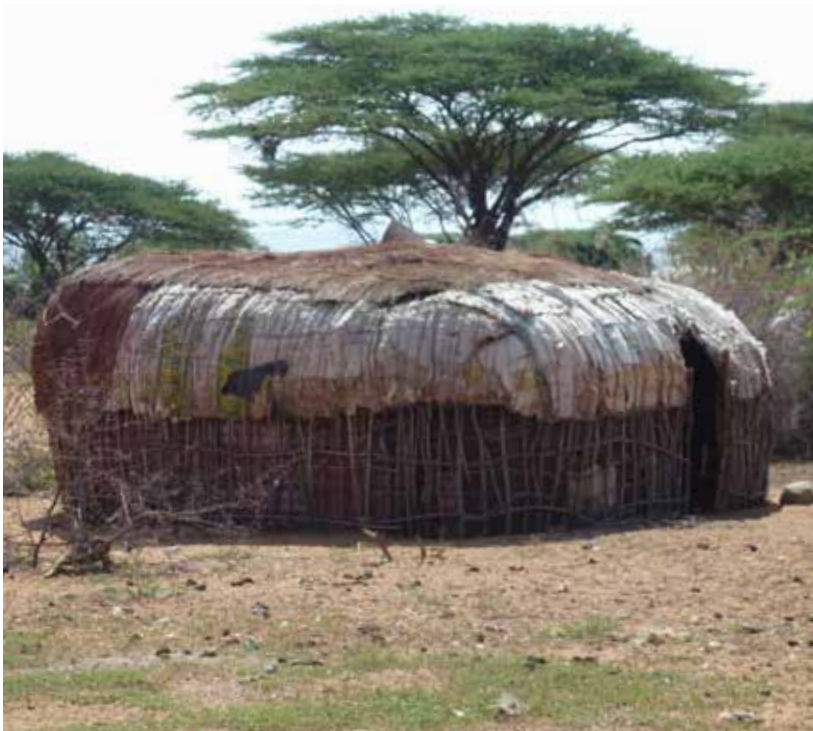
Photo 5: This house, in addition to cardboard boxes, has proper mats (Rendille dulbe , Samburu suut ) as a cover.
