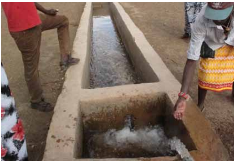
Photo 4: The cement trough is filled by the water pump.
