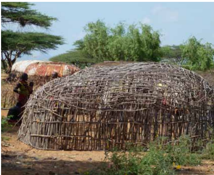
Photo 8: A house under construction
