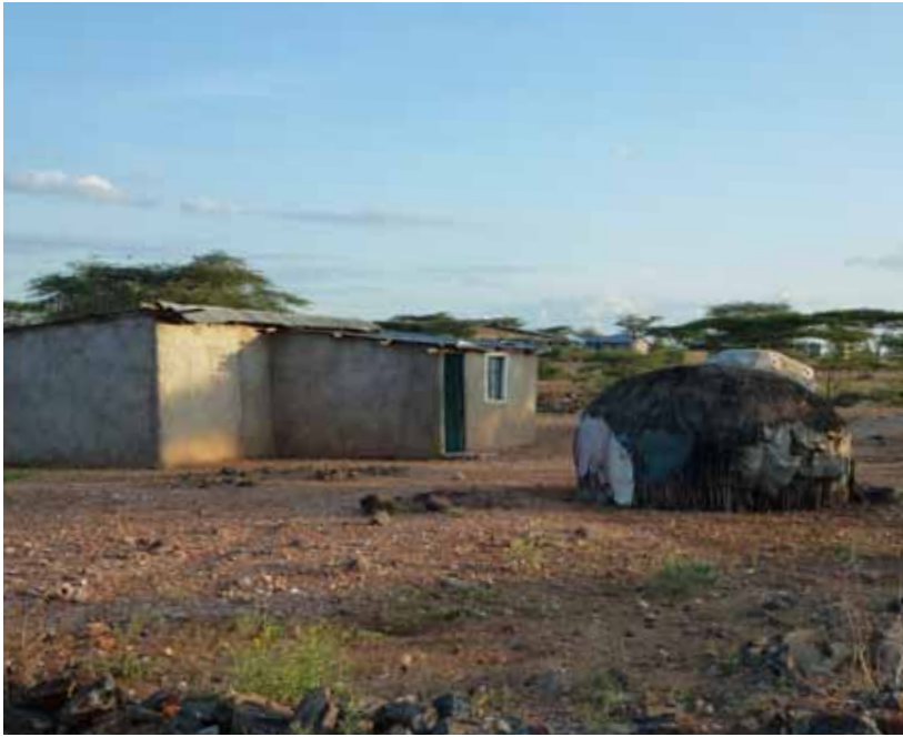
Photo 4: A semipermanent house with a wooden frame filled with stones, covered with cement plaster, and corrugated iron roofing. Note the Rendille style house in the same compound.
