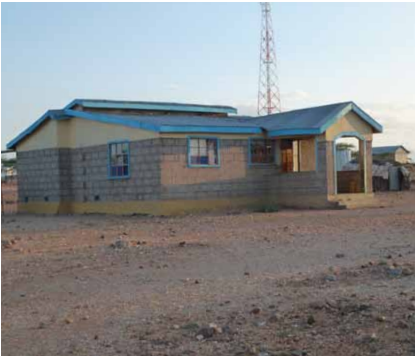
Photo 3: One of the more elaborate permanent houses built with cement blocks with corrugated iron roofing. 20140425
