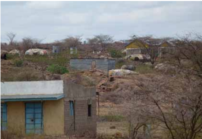
Photo 2: A mixture of houses built of cement blocks, sticks and cardboard boxes and corrugated iron sheets east of the highway.
