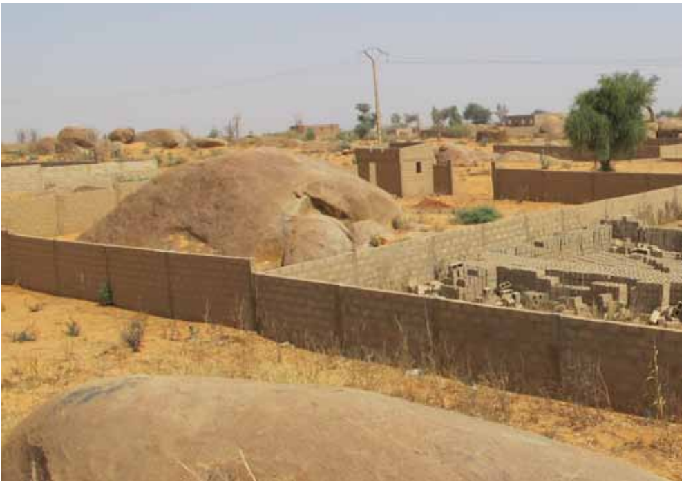
Photo 147: The landscape around Zinder is characterized by rock formations. Here, a plot is dominated by a huge rock, which in a first step has been enclosed by walls. In a second step, the rock will be broken down and the material used for construction. Zinder
