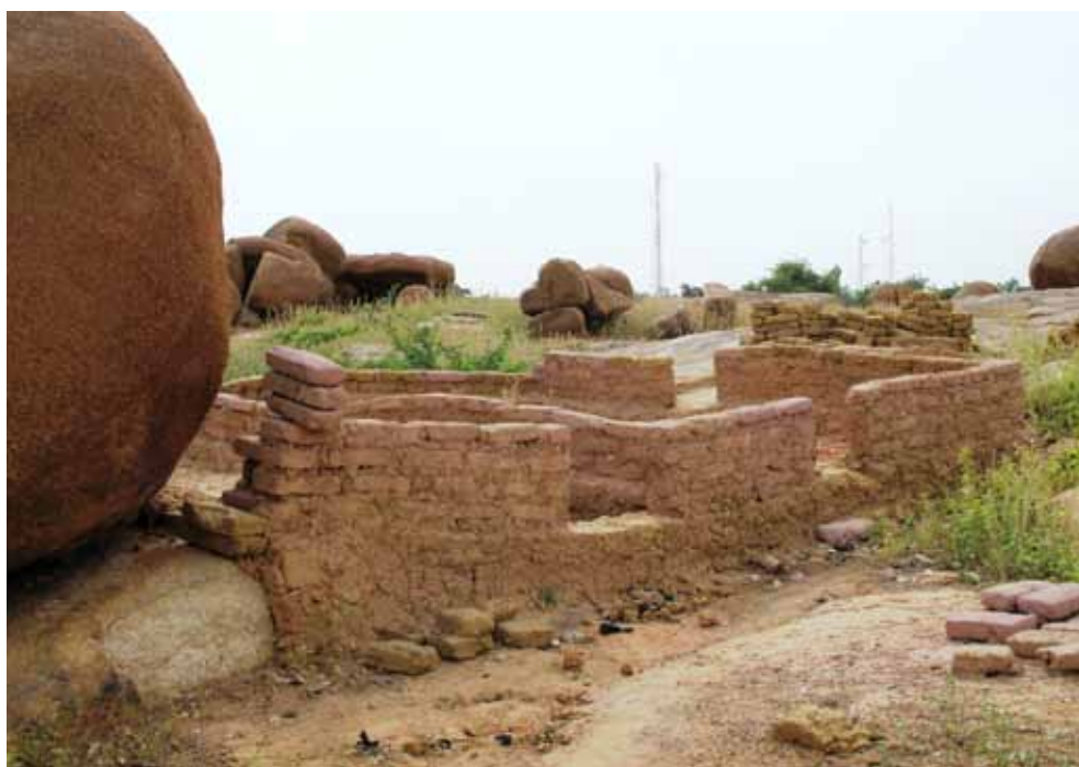
Photo 149: ... The less well-off secure their land claims with simple mud brick walls, which may be erected directly on the rock, sometimes even without levelling the ground. Zinder (F. KÖHLER, 2011)
