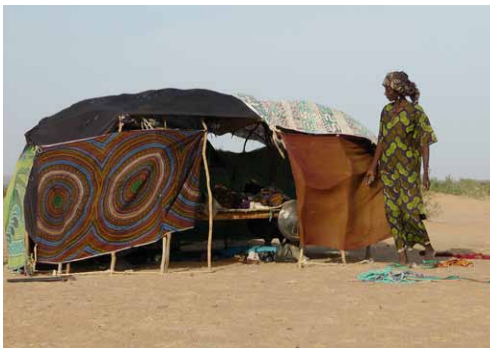
Photo 88: ... During the hot dry season, only a light cover of cloth is preferred, which allows for the circulation of air. Koutous region (F. KÖHLER, 2011)
