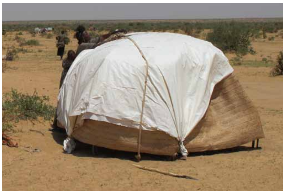
Photo 84: ... During the rainy season, an additional layer of plastic tarp protects the shelter against the rain. Koutous region (F. KÖHLER, 2011)
