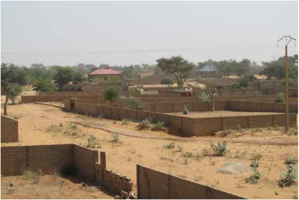
Photo 146: Construction sites mushrooming in the outskirts of Zinder.
