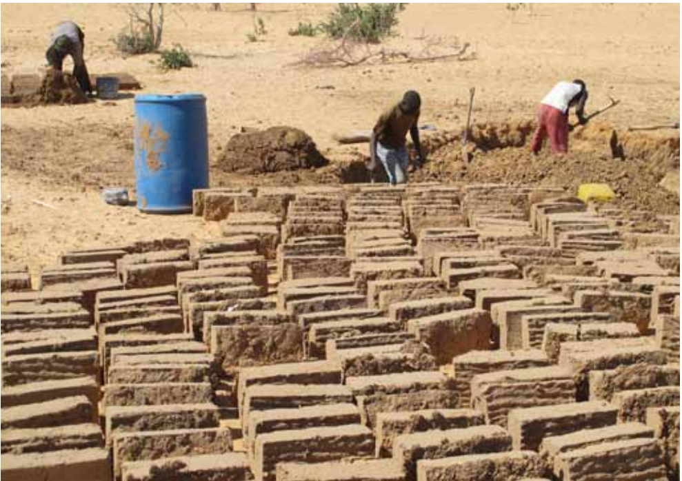
Photos 159–160: The building material of the local construction initiatives are generally mud bricks and hence ephemeral. Salaga, Damergou region (F. KÖHLER, 2011)
