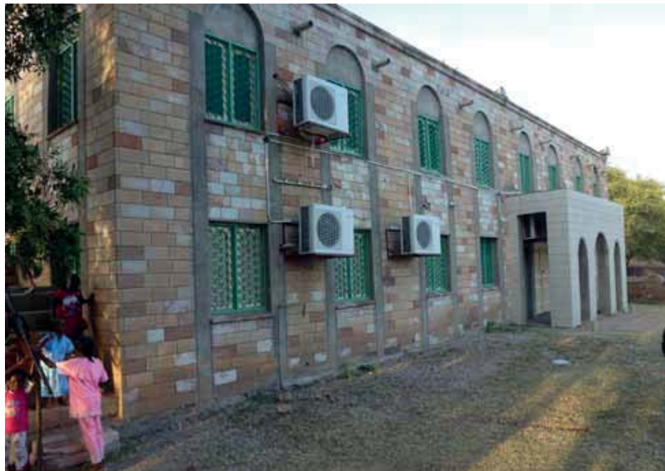
Photo 3: The Central Mosque in Wad Haashim
