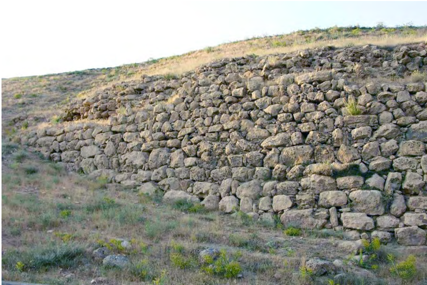
Figure 14.4: Sustaining wall of the “Semiramis Canal,” built by King Minua, south of Van
