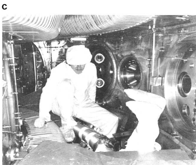
Fig. 69: a) poloidal view of ASDEX with the new divertor target plates. b) 1. coil protection shield (top) and 2. target plate (bottom). c) installation of the lower inner coil protection shield.
