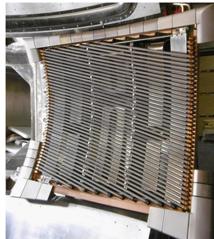
Fig. 7: First antenna during trial installation
