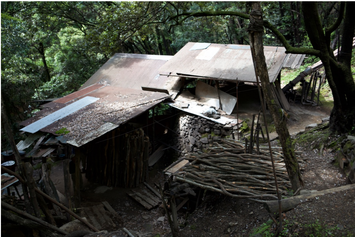
Photo 2: Hara's kiln viewed from above. The main chamber is located under the roof at right. The extended chimneys appear on the far right of the photo; the mouth of the kiln faces downhill, and the area from which it is loaded, monitored and unloaded is located underneath the roof at center. Lengths of oak are lying ready for firing; some will have to be straightened before they can be loaded into the kiln. (photo by the author)
