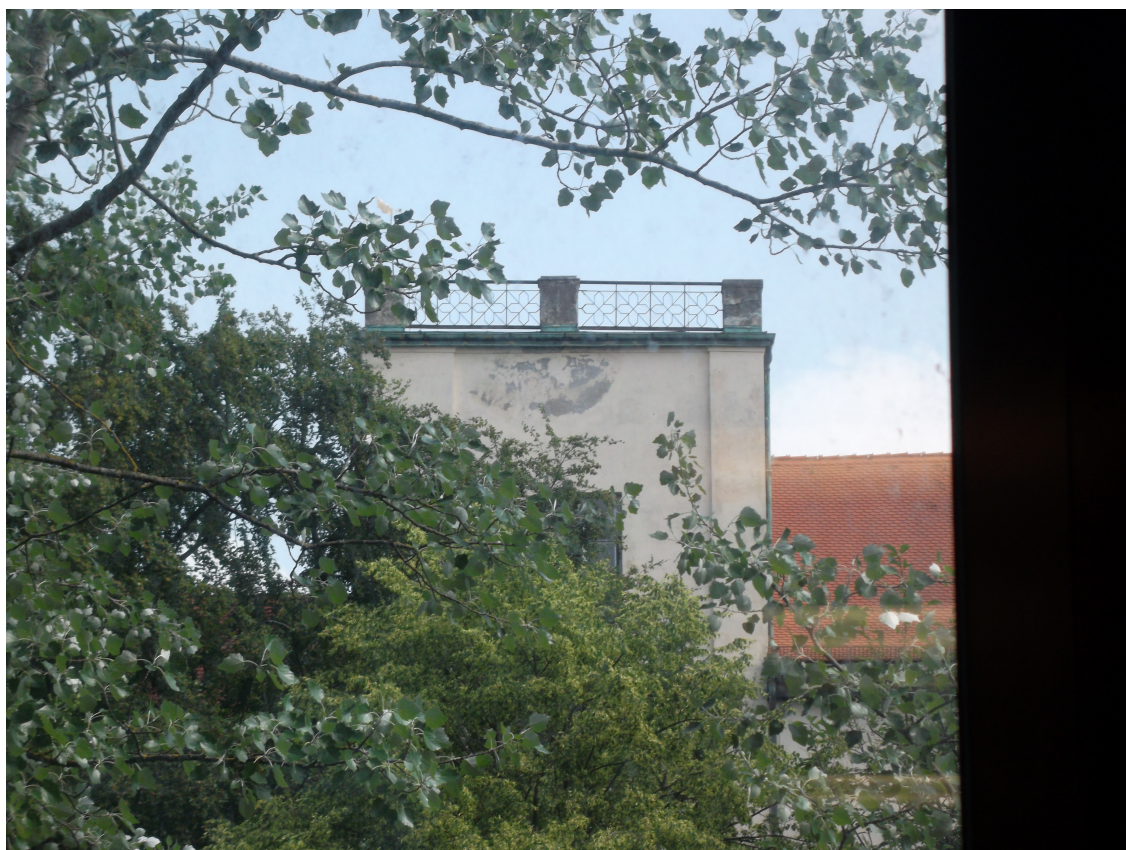
Figure B.1.: Focused camera with view on the balcony bars on the top of the university tower.
