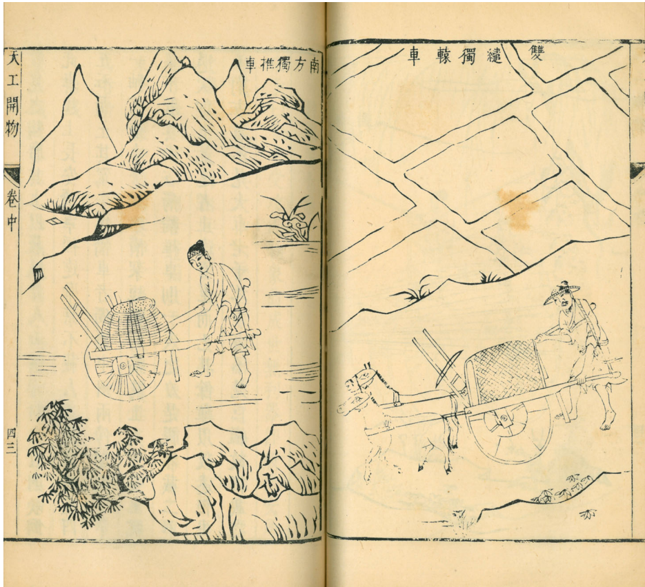
FIG. 3. Left, a single-wheeled cart pushed by one person employed in the south; right, a single-wheeled cart pushed by one person and drawn by two donkeys. (Song Yingxing, Tian-gong kaiwu , 2:42–43.)
