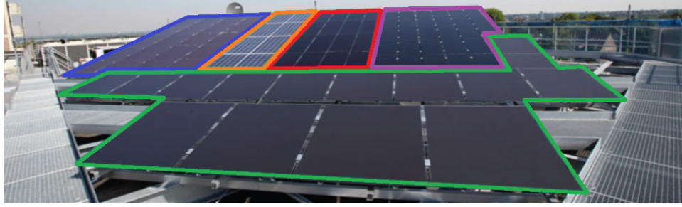
FIG. 1. Overview of the PV site in Mülheim an der Ruhr. Panels highlighted according to the type: \mu\text{m-Si} (green), CdTe (purple), CIGS (blue), poly-Si (orange), and a-Si (red).
