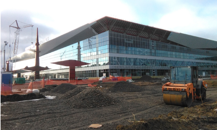
Fig. 2.6. New airport terminal at Yemel'ianovo (Krasnoïarsk) under construction for the Universiade 2019. Photograph by Dennis Zuev, 21 September 2017, CC-BY.
