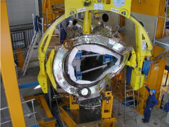
Fig. 1. Threading a non-planar coil across a segment of the plasma vessel
