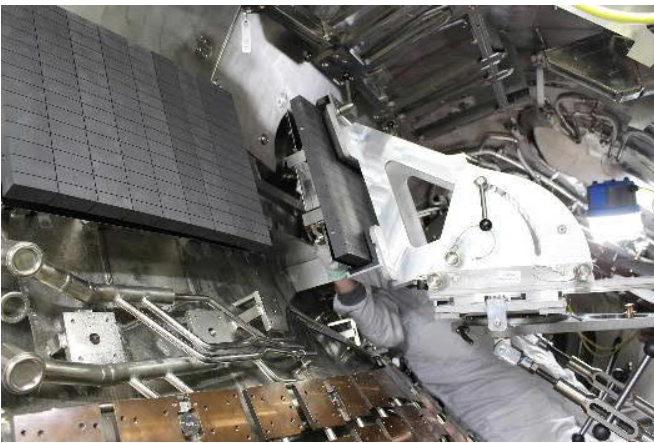
Figure 7: Installation of vertical target modules by means of a positioning device.
