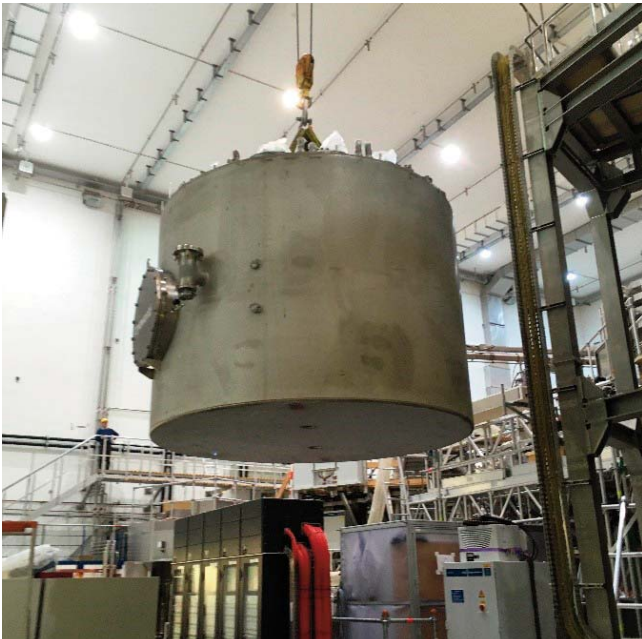
Figure 14: Transport of the valve box inside the torus hall.
