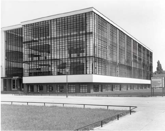
FIGURE 1C: FACADE OF THE BAUHAUS DESSAU WORKSHOP WING, SHOWING THE CURTAIN WALL
