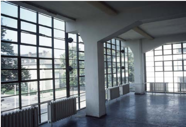
Note the extensive radiators exposed to the glazing.
