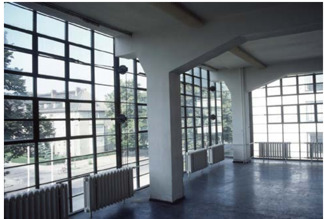
FIGURE 2A: A TYPICAL WINDOW WALL OF THE WORKSHOP WING OF THE BAUHAUS DESSAU BUILDING
