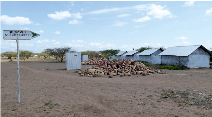
The construction of permanent shelters in Kalobeyei, 27 July 2018. (Photo: Stefan Millar)
