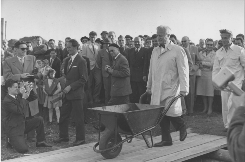
Fig. 1 William Sterling Cole, the first Director General of IAEA, pours the first load of concrete into the foundations of the new laboratory to inaugurate construction on September 28, 1959. The laboratory began operating two years later. (Courtesy of the IAEA Archives)
