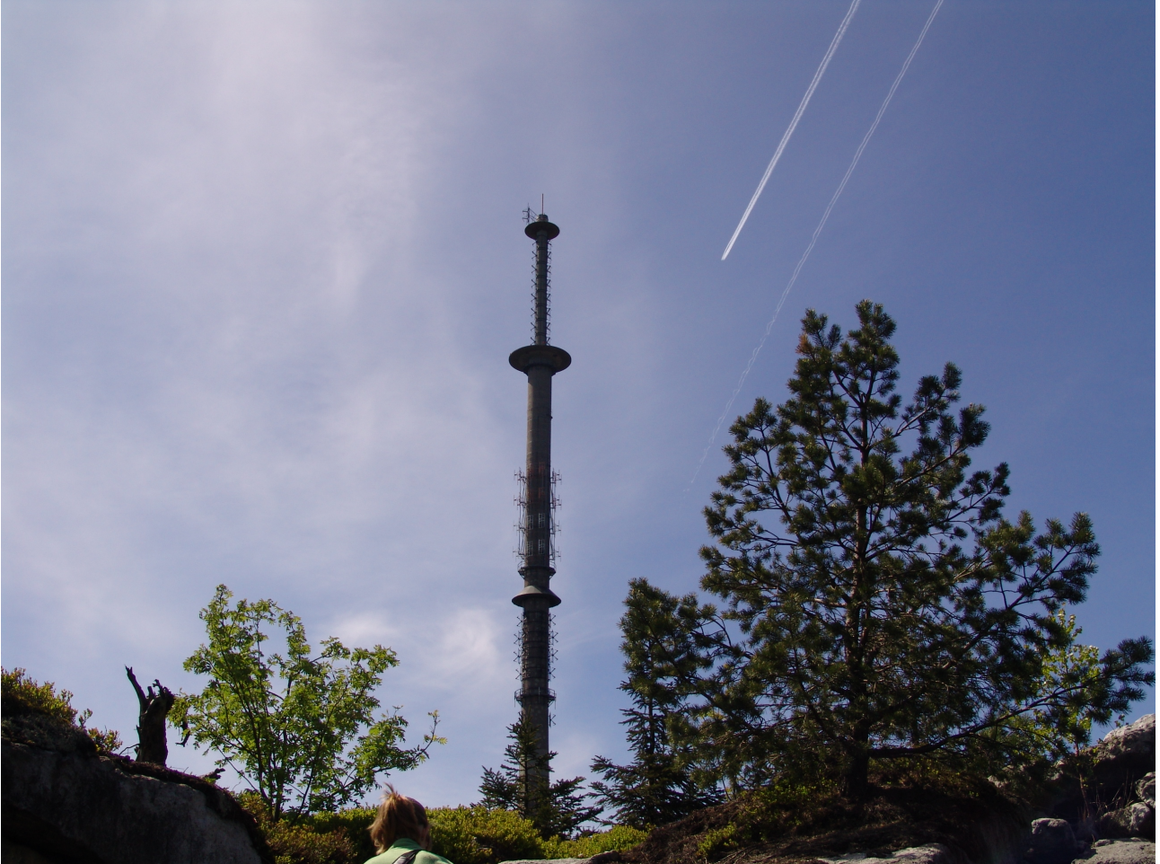
Figure 24: Ochsenkopf communication tower, Germany
