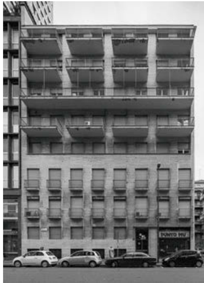
176 Mario Asnago and Clau- dio Vender, house at the Viale Tunisia, Milan (Italy), 1935–36.
