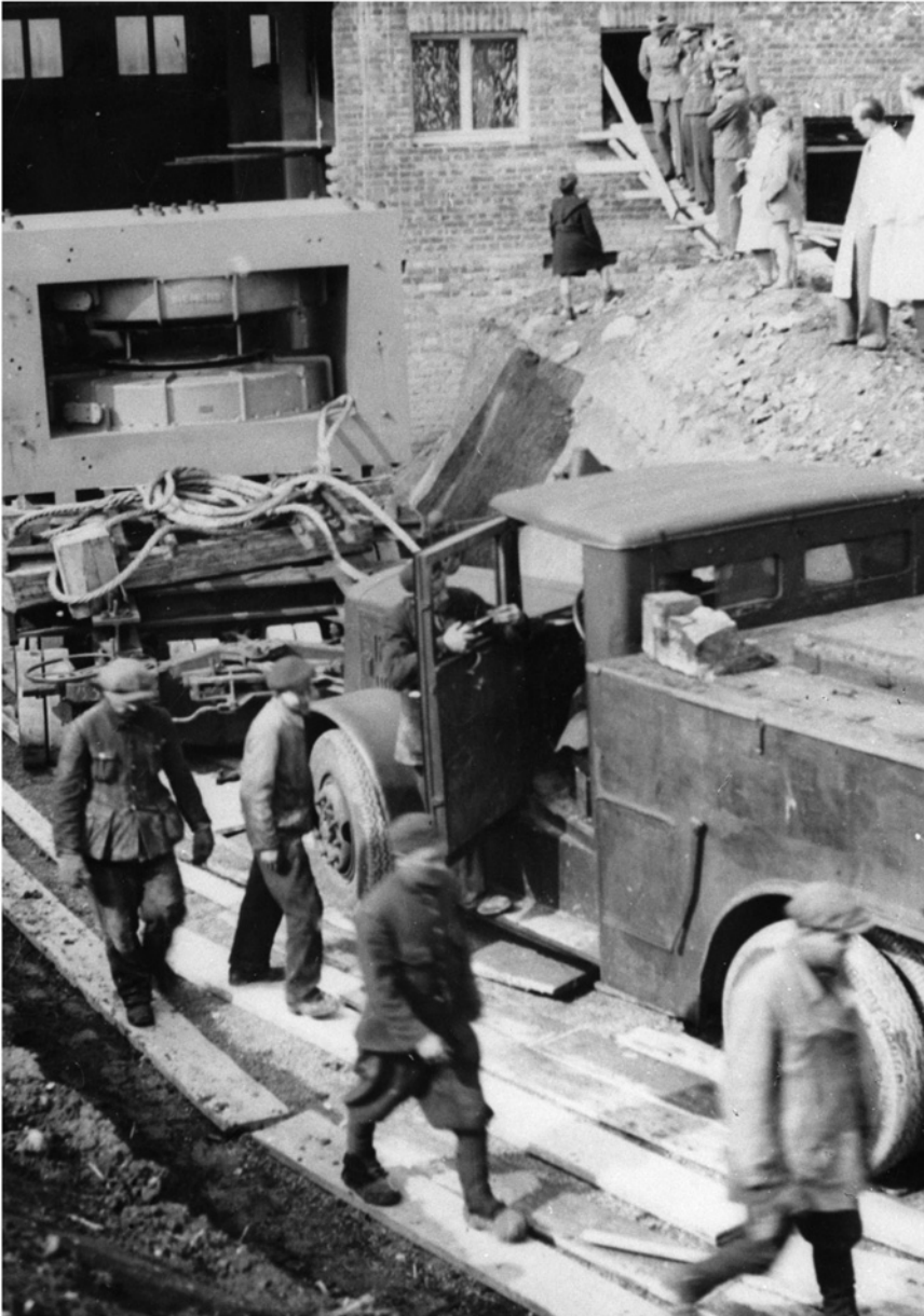
ILLUSTRATION 47 Kaiser Wilhelm Institute for Medical Research, Heidelberg. The cyclotron magnet ready for installation, 1943. Russian prisoners of war were employed for transport and installation operations.
