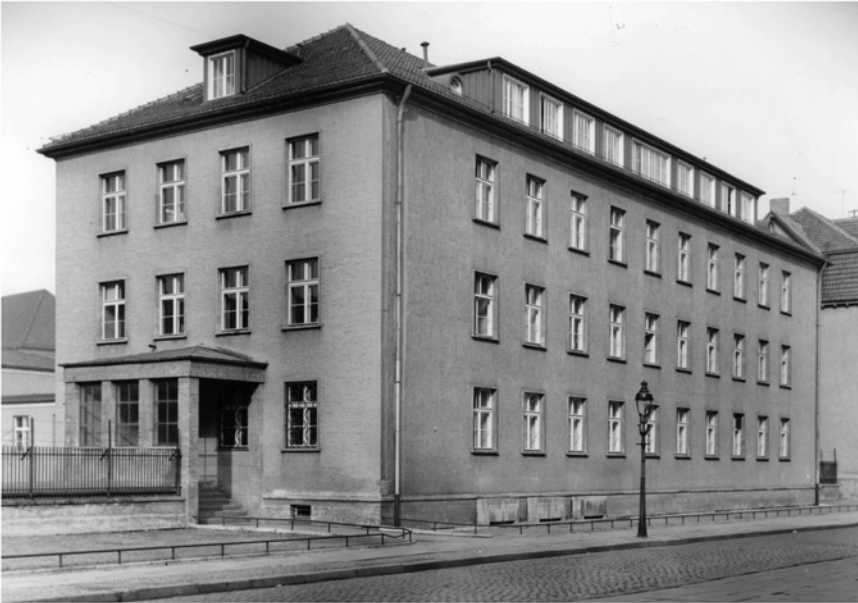
ILLUSTRATION 4 The Max Planck Institute for Physics in Göttingen on Bunsenstrasse, housed since the summer of 1946 in Building No. 10 of the Aerodynamics Research Institute (AVA), which formerly contained a cooling tunnel.
