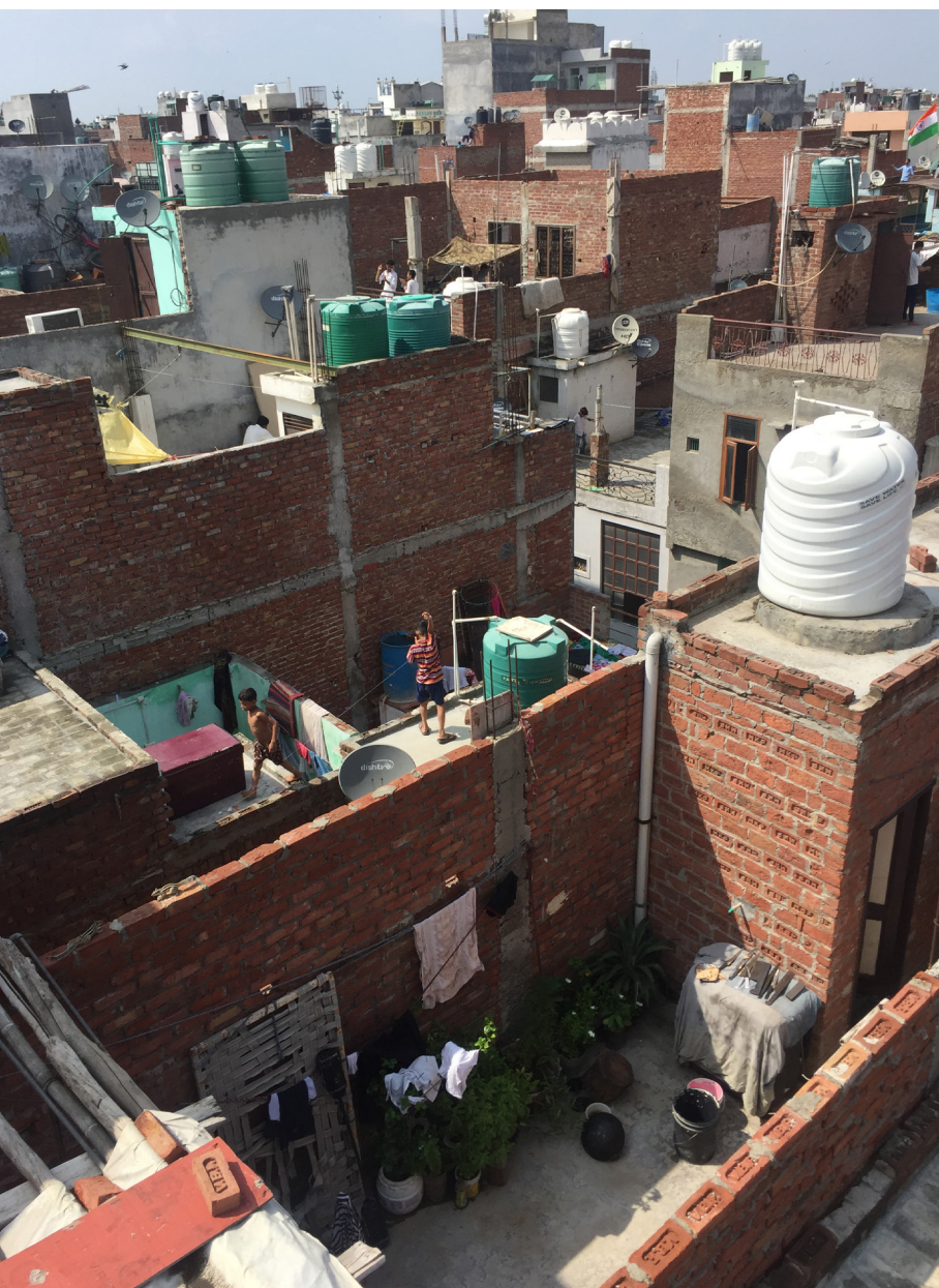
Fig. 7. Life on the rooftops is a testimony to the inhabitants' desire for space and air. Kabadabad, August 2019.
