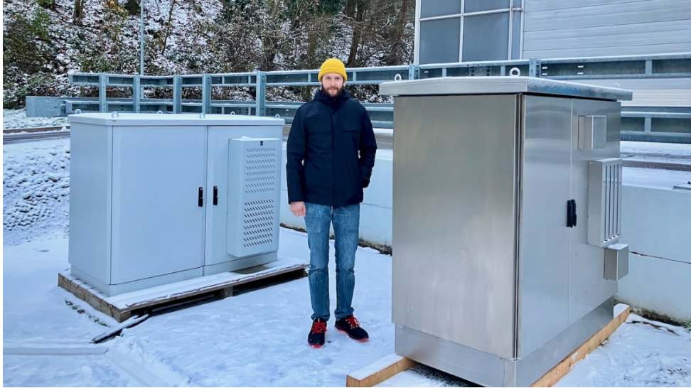
Figure 48 Two prototype DAQ nodes operating next to the SWGO test tank at MPIK, Heidelberg. Left: Rittal CS TopTec cabinet with Blue e+ KG chiller; middle: Myself for scale (~1.9 m high); right: custom-made Häwa cabinet and Seifert air-to-air heat exchanger unit.
