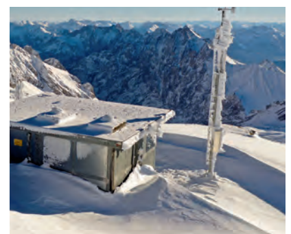
Fig. 29: Measurement hut on top of the “Schneefernerkopf” 2.875 m above sea level (see also Fig. 28)
