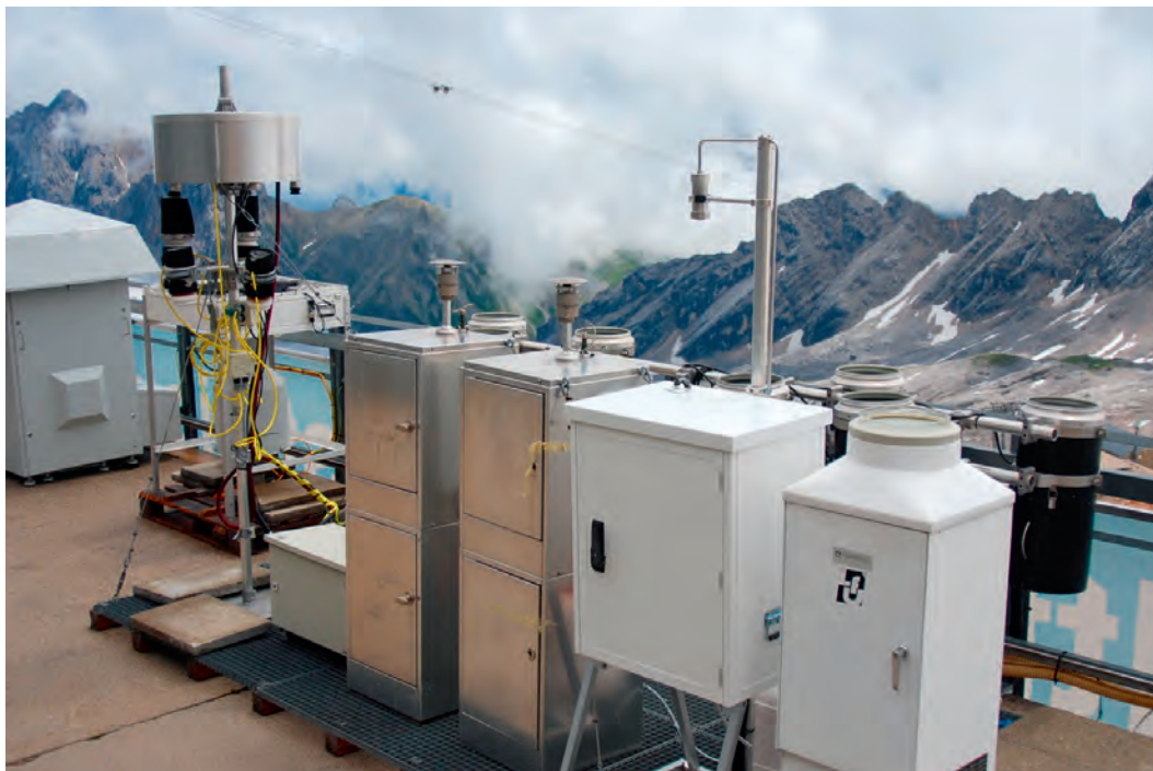
Fig. 1: Measurement equipment at the UFS for sampling ambient air and deposition for the detection of persistent organic pollutants. Picture: KF, LfU
