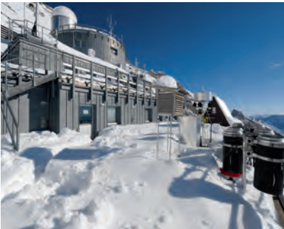
Fig. 32: View of the UFS building and some measurement devices
