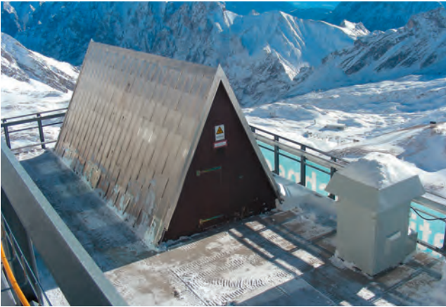
Fig. 11: Instrument shed on the measurement terrace of the UFS housing the Extended-Range Bonner Spheres Spectrometer of the HMGU (see also Fig. 5).
