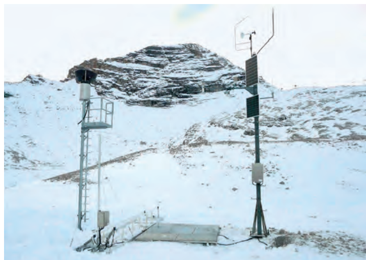
Fig. 8: Meteorological station at central Zugspitzplatt (2420 m a.s.l.), operated by the Bavarian Avalanche Warning Service and the authors on behalf of the Environmental Research Station Schneefernerhaus. It is equipped with sensors for the determination of standard meteorological and snow parameters. The measurement data is recorded and transferred to the Alpine Environmental Data Analysis Center (AlpEnDAC, www.alpendac.eu ), where it is publicly available (Photo: F. Bernauer, 2012-11-08).
