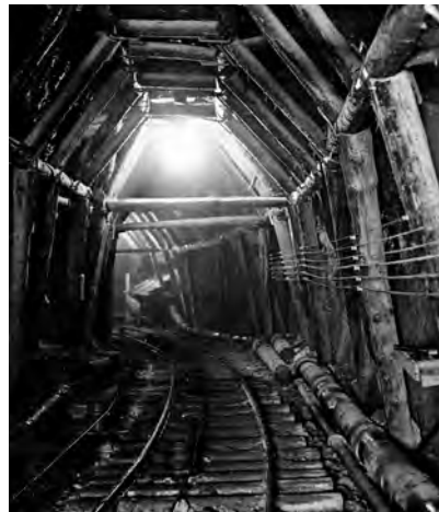
Fig. 11: Wooden shuttering in the tunnel during construction in 1929
