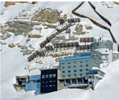
Fig. 33: View from the Zugspitzplatt to the UF building with the rockfall and avalanche protection system
