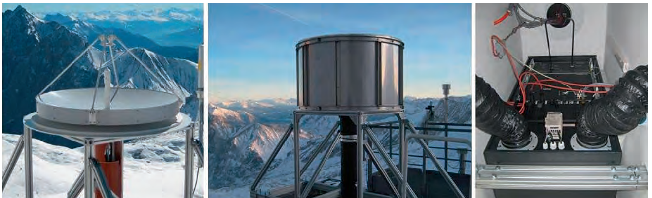
Fig. 2: Installation of the MIRA36 cloud radar at Umweltforschungsstation Schneefernerhaus. Left: antenna of Casagrain type during the installation phase with parabolic dish, feed horn in the center and sub-reflector at the top. Center: antenna with clutter fence. Right: radar transmitter and receiver within the suspended ceiling of Wechselnutzlerlabor. Photos by M. Hagen.
