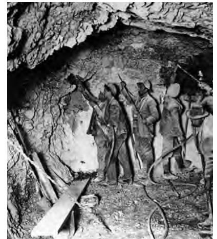
Fig. 12: Workers during excavation work on the Zugspitze tunnel for the planned cogwheel railway
