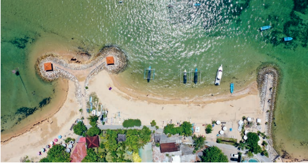
Shoreline fortification after beach replenishment in Sanur, Denpasar.
