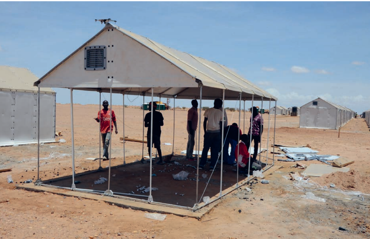
Day labour migrants assemble IKEA's "Better Shelter" huts in the Sahara to house Sudanese refugees who had fled the Libyan civil war. The refugees later criticized them for not being adapted to the heat and dust. Agadez, Niger, 2018.
