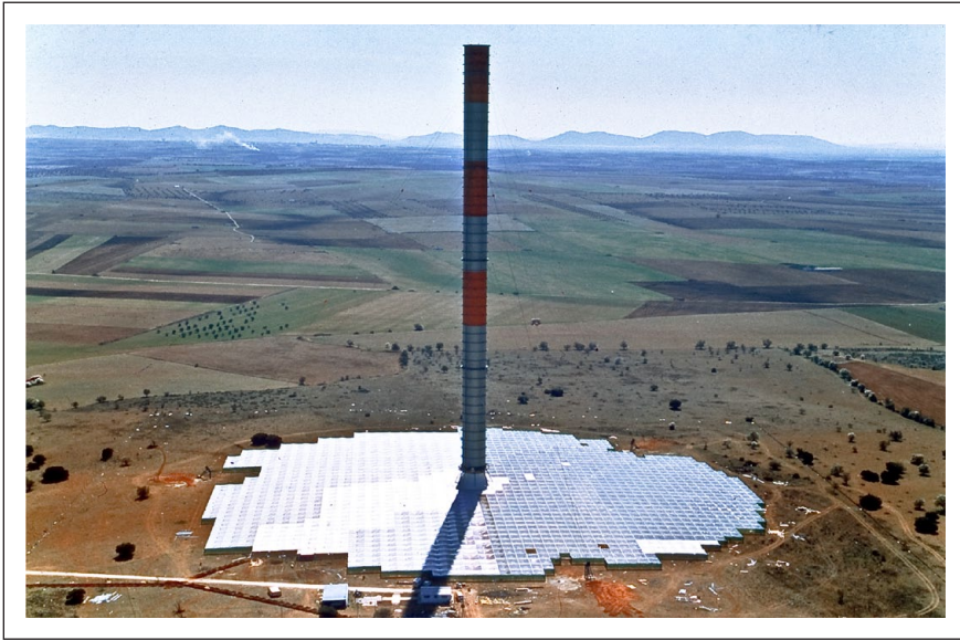
Figure 4. The solar updraft demonstration facility at Manzanares, Spain, built in 1982. Heat from solar radiation causes an updraft from the structure's perimeter, which exits through the chimney. Image © sbp sonne.
