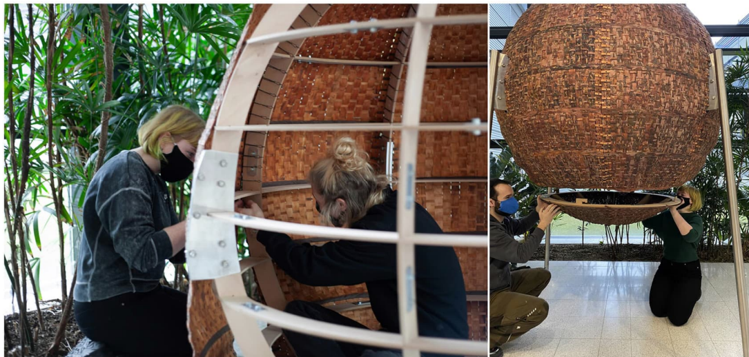
Figure 5.4.9: Final connection of bark skin to the inner structure. Closing the sphere. The cap is hung on the body of the sphere with a bayonet lock.
