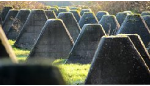
Figure 1 . These now unnecessary anti-tank obstacles were part of the Westwall, a National Socialist defense line on the French and German border.
