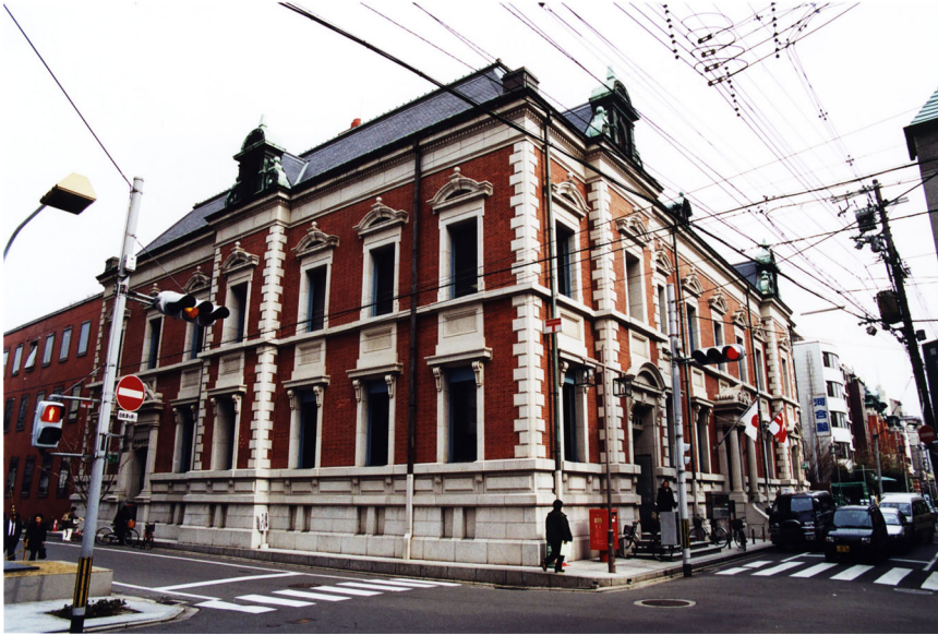
Figure 3. Prewar post office building on Sanjō Street. (Photograph by the author.)
