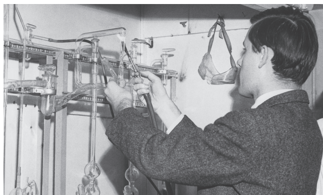
Figure 4. The author preparing an evacuated pyrex chemiluminescence cell. Safety considerations did not get top priority at the time: a laboratory coat or safety glasses, although available (see photograph), were not always used.
