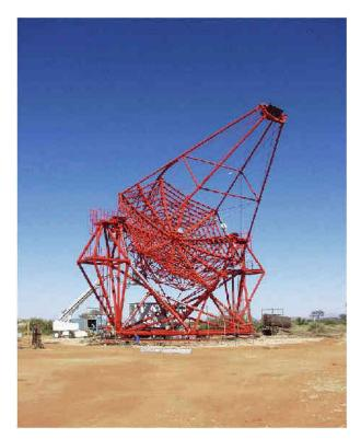
Fig. 24. Steel frame of the first H.E.S.S. telescope. Rotation around the vertical axis is on a circular rail of  $\sim 15$  m diameter.
