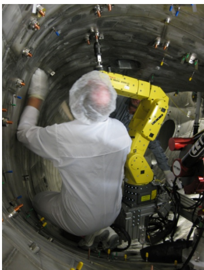
Fig. 5. Installation of in-vessel components.
