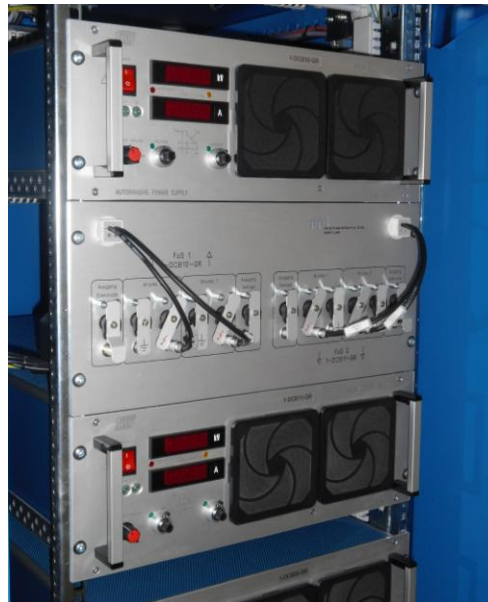
Fig.1 rack showing two converters and the connections to the electrodes, to the test load as well as the grounding bridges.
