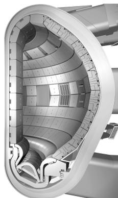
FIG. 1: In-vessel view of ITER. The surface of the main chamber is Beryllium, the material of the divertor (in lower part of the vacuum vessel) is carbon and tungsten. Source:[1], published with permission of ITER.
