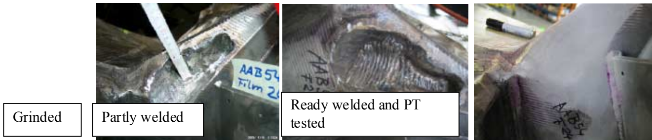
Fig. 9: Repair of a casing defect
